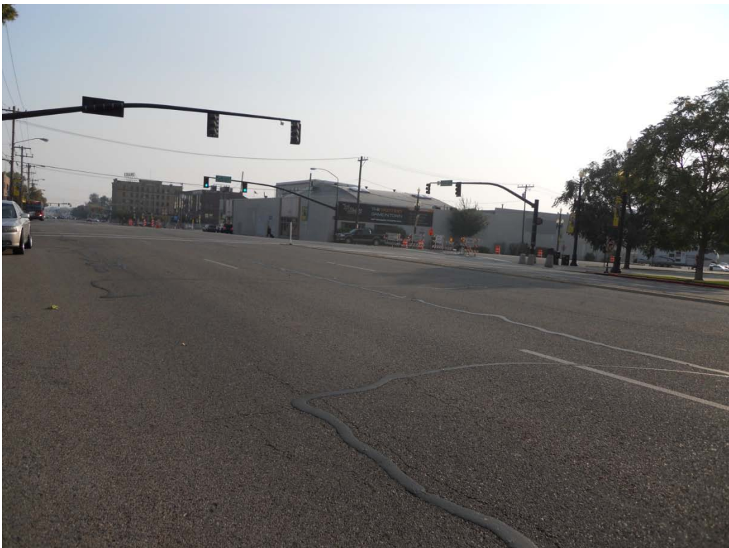
300 West 100 South intersection (looking southwest)
