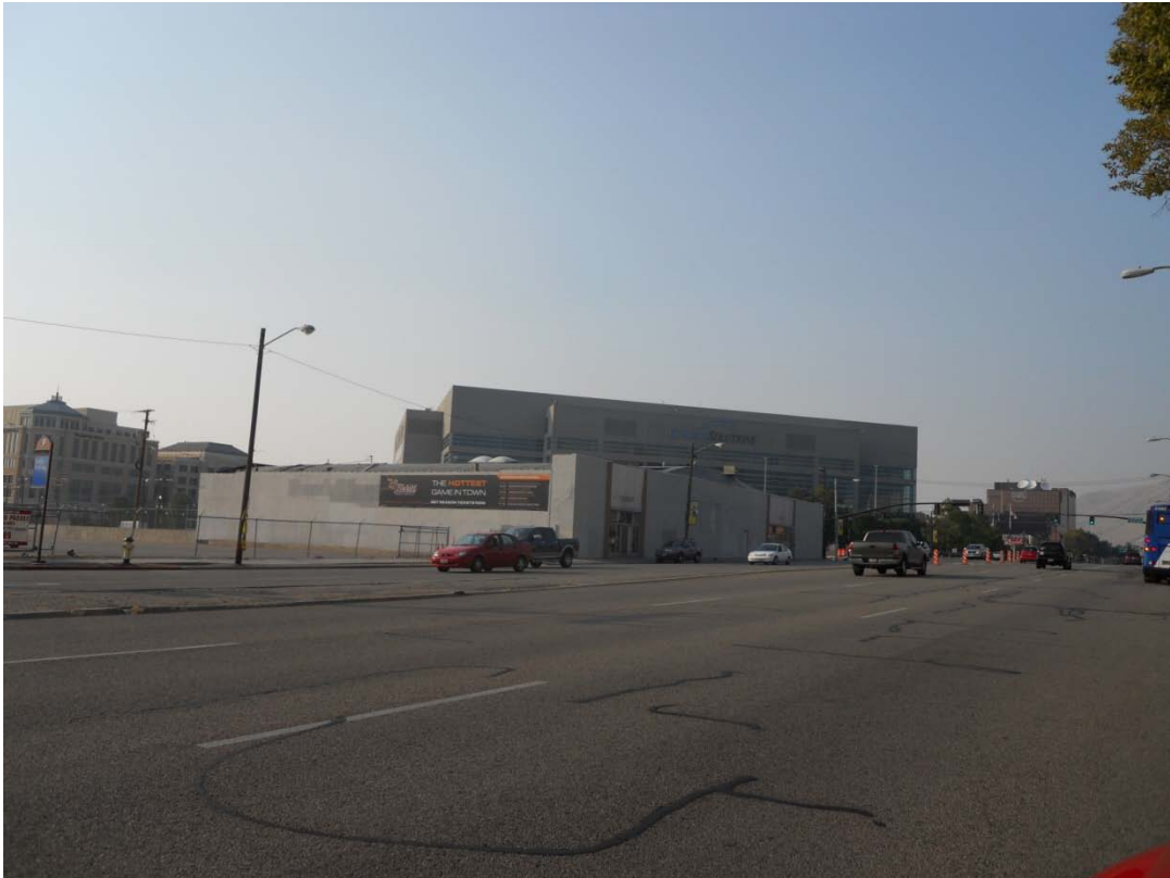
300 West (looking northwest)
